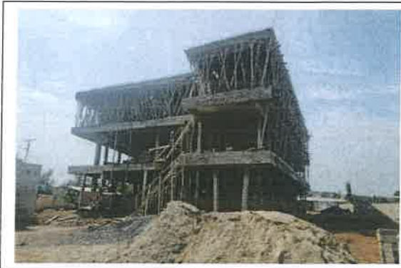
EXECUTION DE LA DALLE R+2
