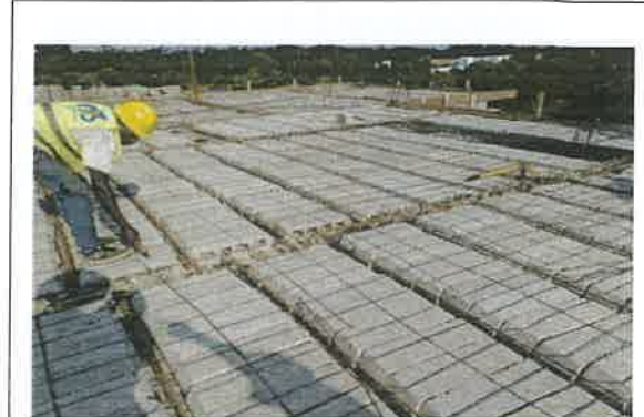
EXECUTION DE LA DALLE R+2
